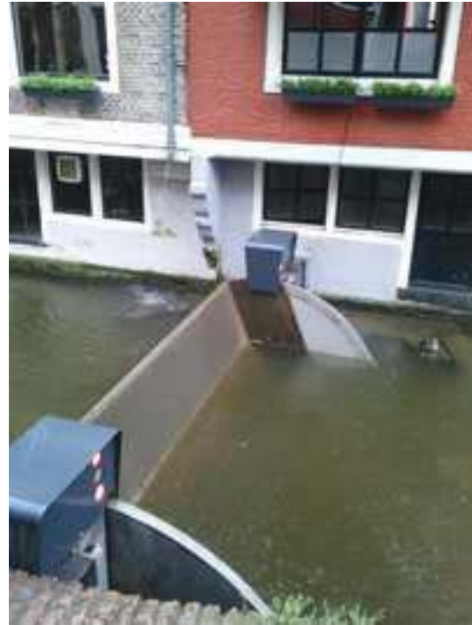
Figure 15: Adjustable weir in closed position
